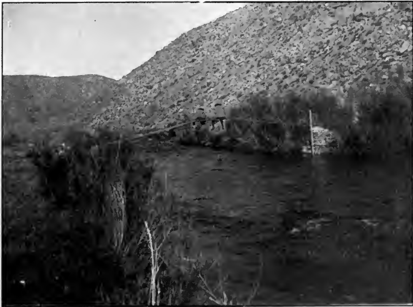
OWENS RIVER GAGING STATION
